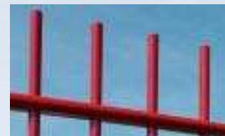
Bars extending from rail Cut straight across
