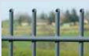
Bars extending from rail Cut off at 45°
