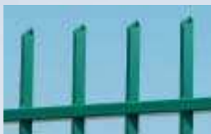
Bars extending from rail Cut off at 45°
