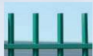
Bars extending from rail Cut straight across
